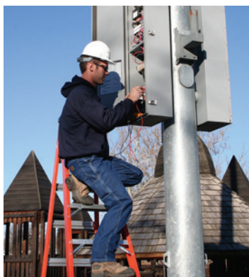
Having major electrical components accessible at ground level avoids hiring a $100/hour crane to replace a $10 fuse.
